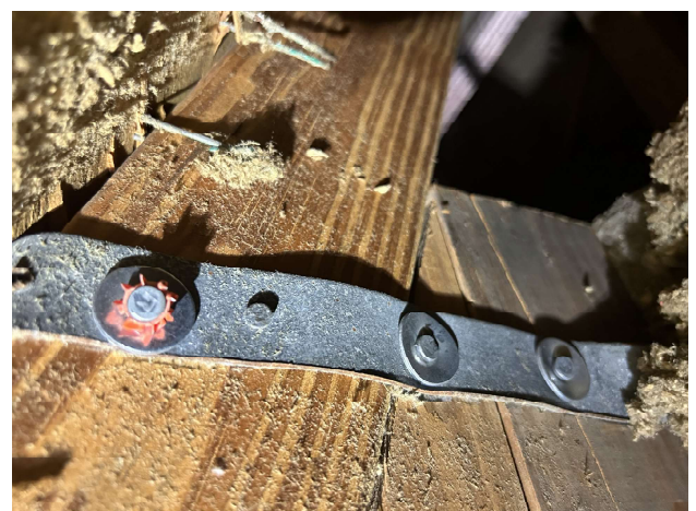
Roof to wall attachment - Clips
