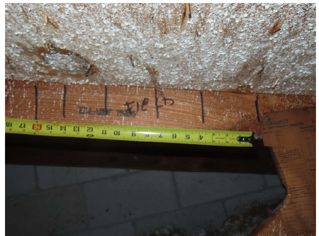
Roof deck nail spacing - Field
