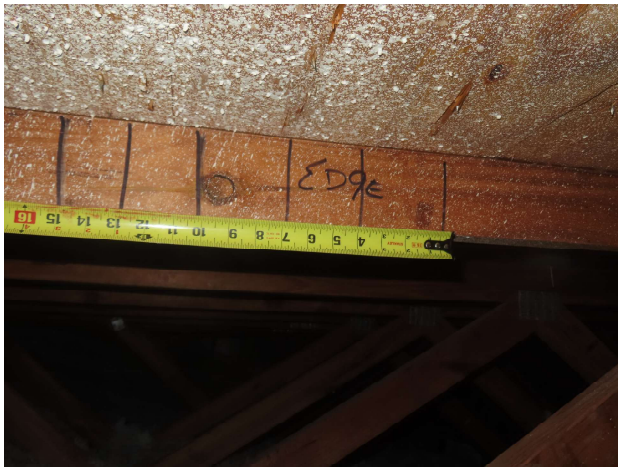
Roof deck nail spacing - Edge
