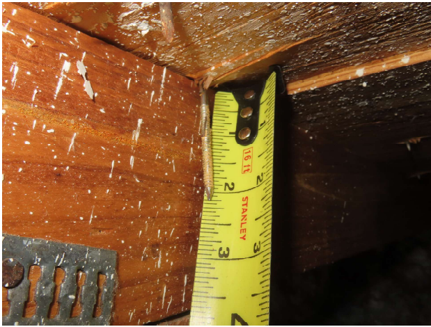
Roof to wall attachment - 8d nails
