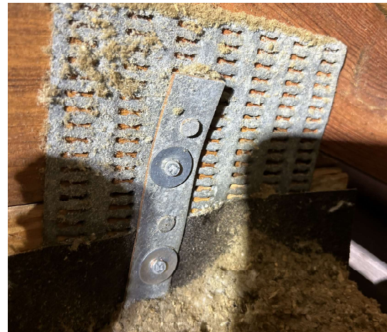
Roof to wall attachment - Clips
